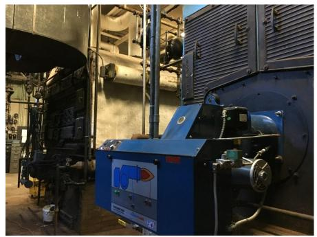
Boiler room – to the left is the older and oil fed boiler, newer gas fed boiler is to the right
