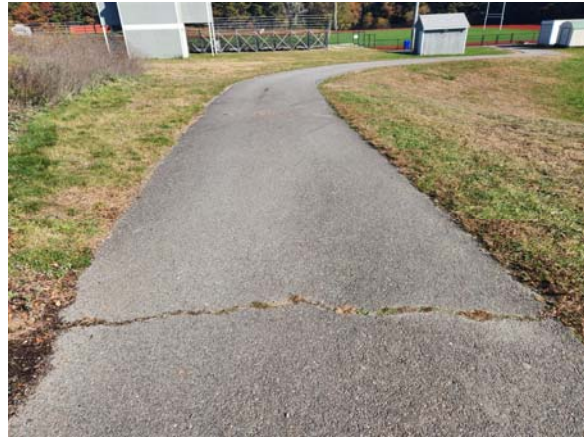
Figure 14 – Sample transverse pavement crack.
