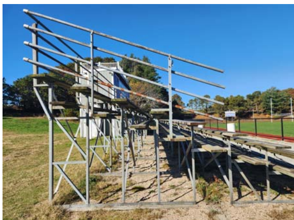
Figure 5 – Bleacher structure fall protection railing.
