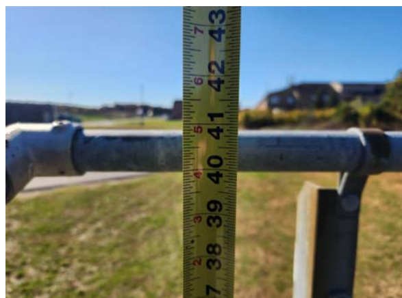
Figure 6 – Bleacher structure fall protection railing measured to be 41-inches from top of the timber seat.
