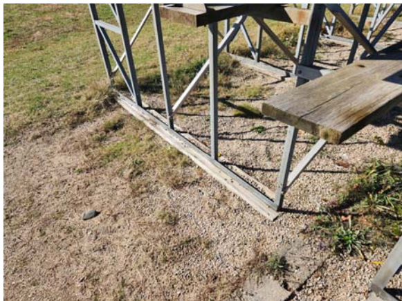
Figure 3 – Bleacher structure timber foundation and gravel subbase.
