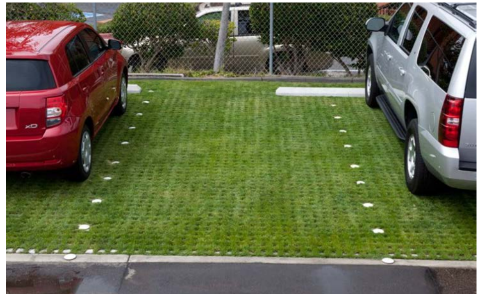
Drivable permeable pavers are an attractive and low-maintenance alternative to asphalt.
