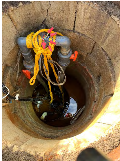
Figure 2-4: Suspected Tidal Inflow MH
