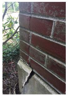
Cracking masonry and foundation wall
