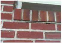
the brick is evident at several locations throughout the façade. The brick façade on the 1959 addition failed and a portion was replaced with textured T-11 exterior plywood siding. Some brick spandrel panels on the 1953 building have been replaced with vinyl siding.
