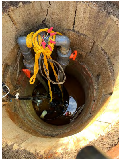
Figure 2-4: Suspected Tidal Inflow MH
