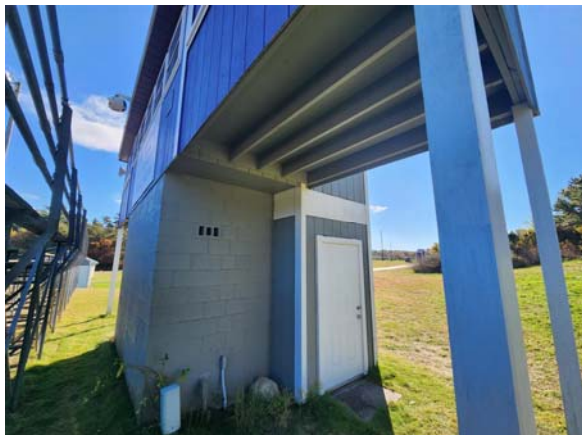
Figure 11 – West underside of press-box building structure.
