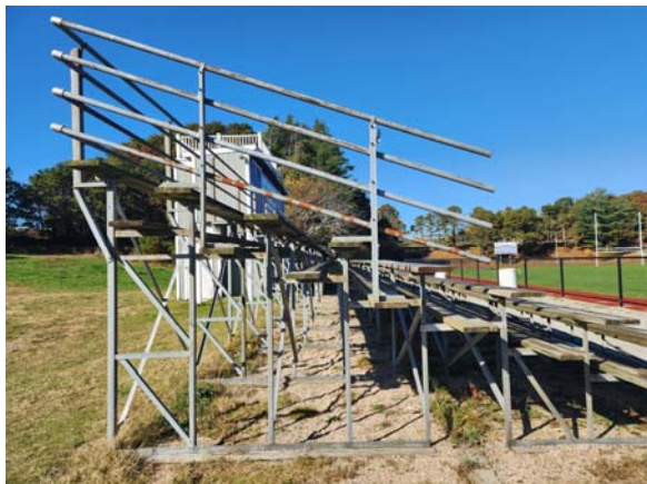
Figure 5 – Bleacher structure fall protection railing.
