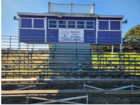
Figure 7 – Front/north side of press-box building structure.
