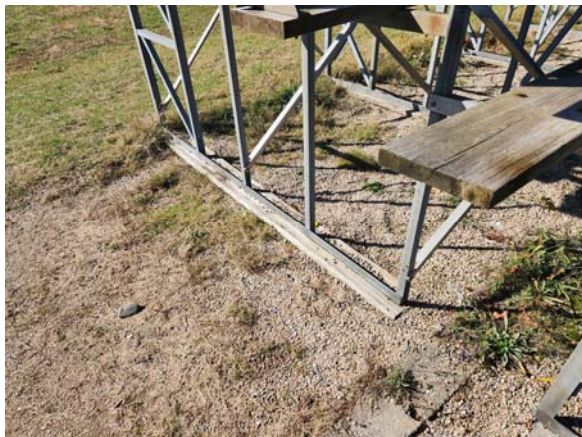
Figure 3 – Bleacher structure timber foundation and gravel subbase.
