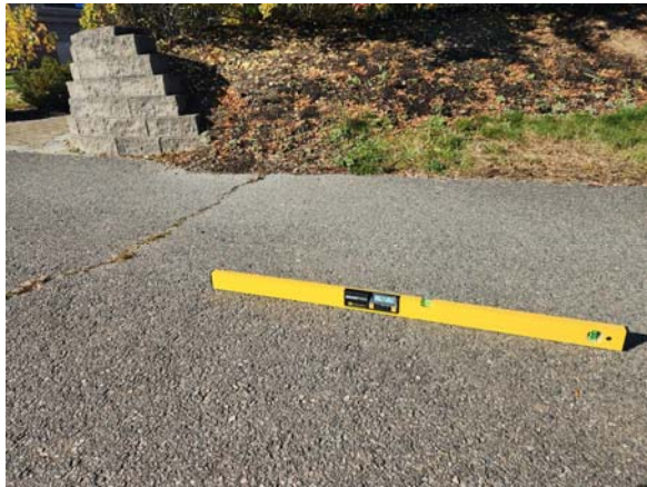
Figure 15 – Sta. 0+50 pavement walkway profile slope.
