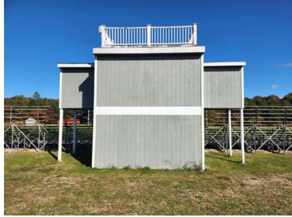
Figure 8 – Rear/south side of press-box building structure.
