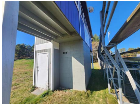
Figure 12 – East underside of press-box building structure.
