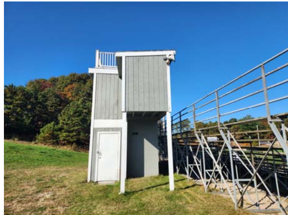
Figure 10 – East side of press-box building structure.
