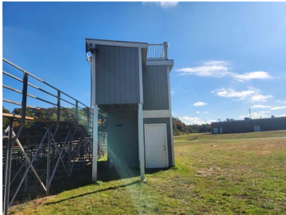
Figure 9 – West side of press-box building structure.
