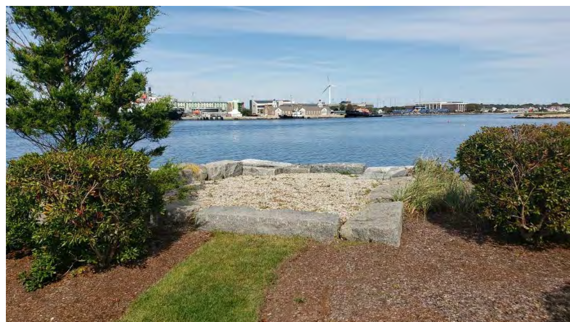
EXISTING BULKHEAD LOOKING NORTH
