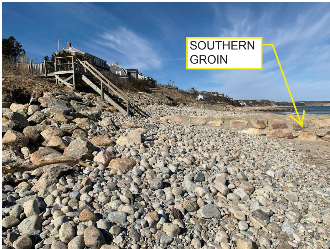
Southern Groin – facing north – fill required on southern side
