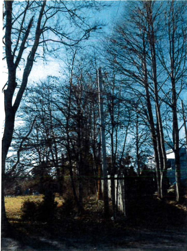
Photo 1: Sample photo illustrating the existing wood pole (to be removed and replaced).
