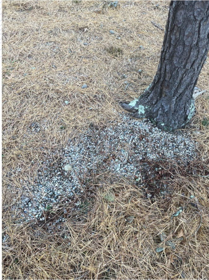
Picture 2 – Existing condition of one of the trees on the bank – significant portions of the bank have peastone, pavement and moss areas – no presence of stabilizing vegetation.
