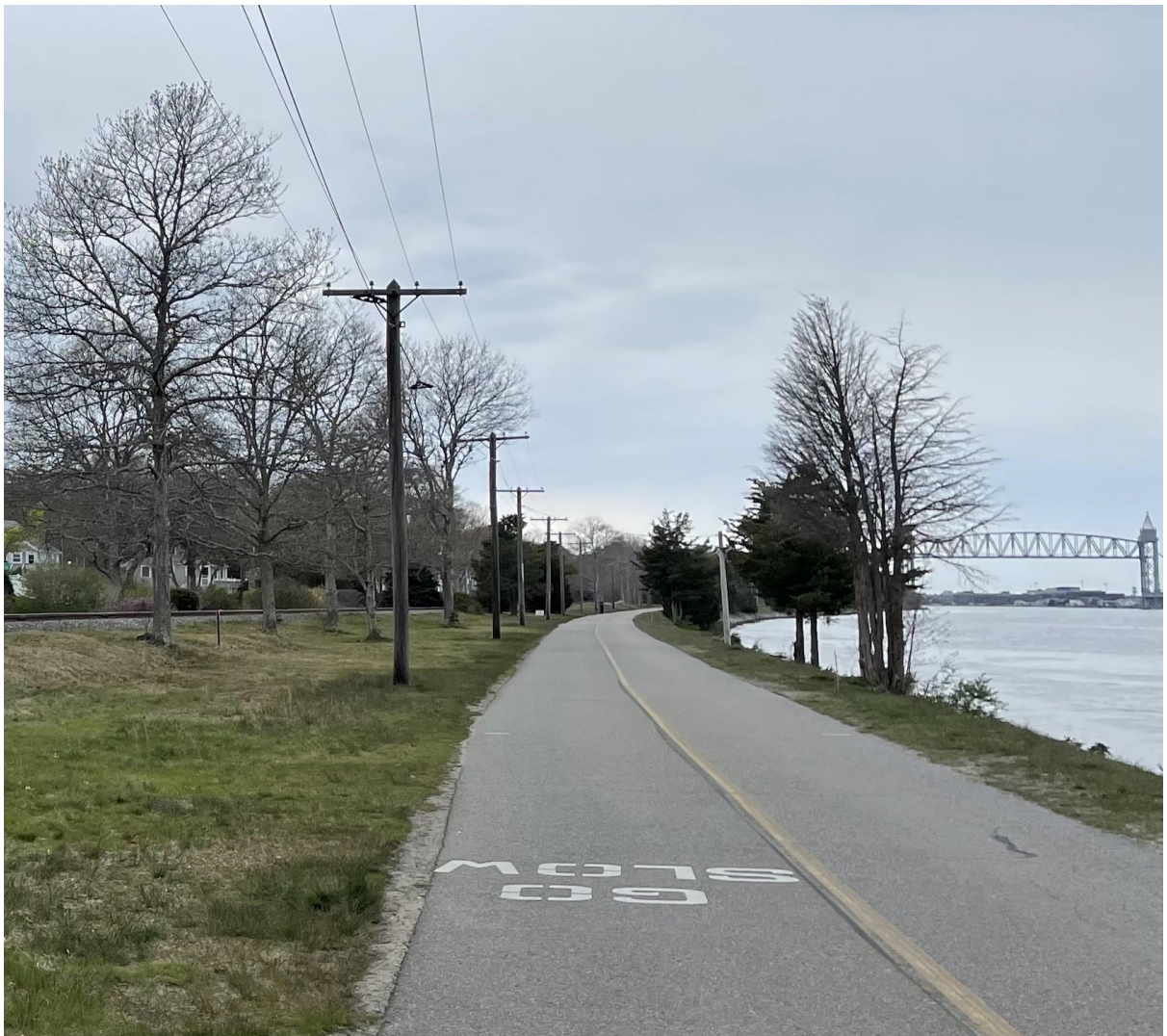
Cape Cod Canal Bikeway, Cape Main Line, and Cape Cod Canal Railroad Bridge
