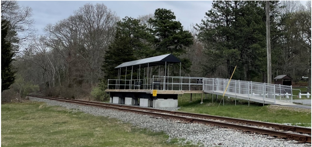
Existing platform at Bourne
