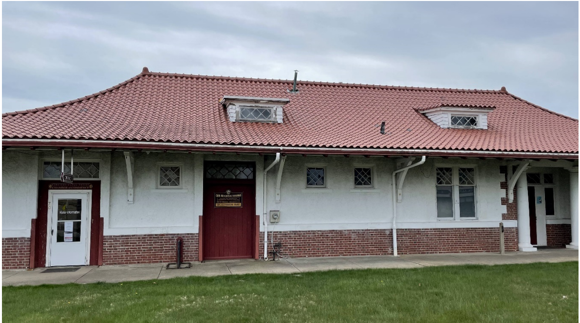
Existing station building at Buzzards Bay
