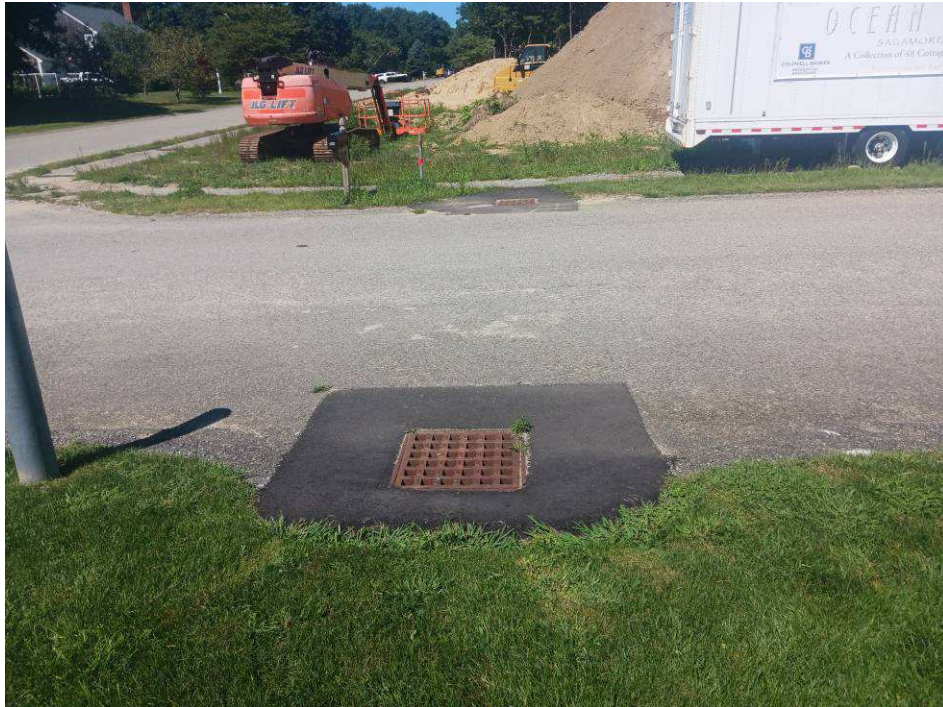
Figure 3 – Entrance Catch basin on Wildwood Lane
