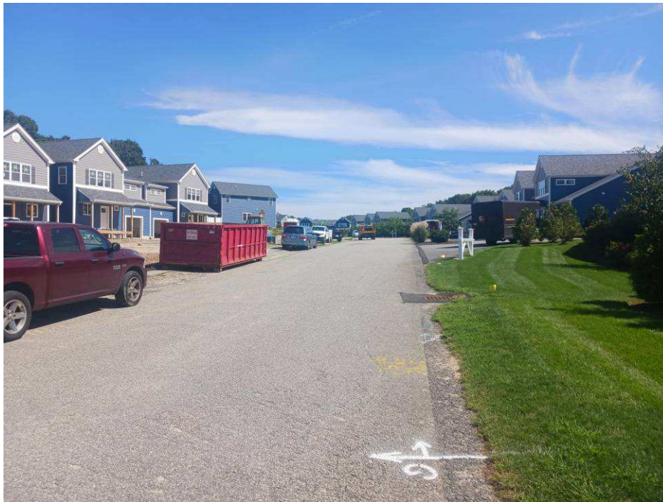
Figure 4 – Looking West down Wildwood Lane showing catch basins
