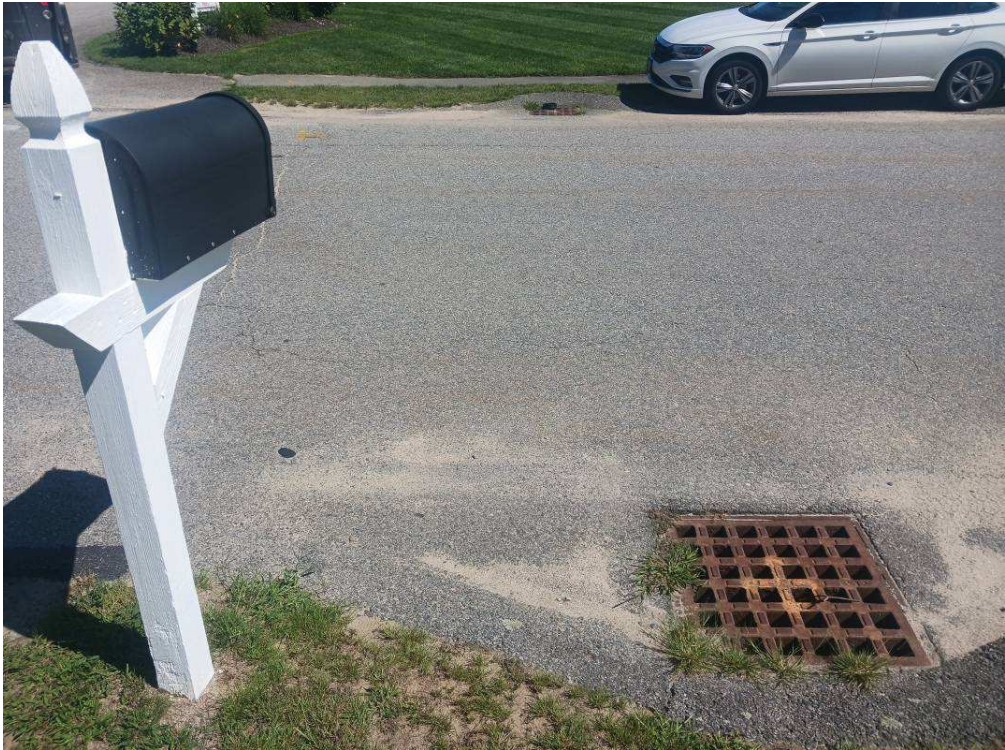
Figure 2 – Catch basin along Wildwood Lane
