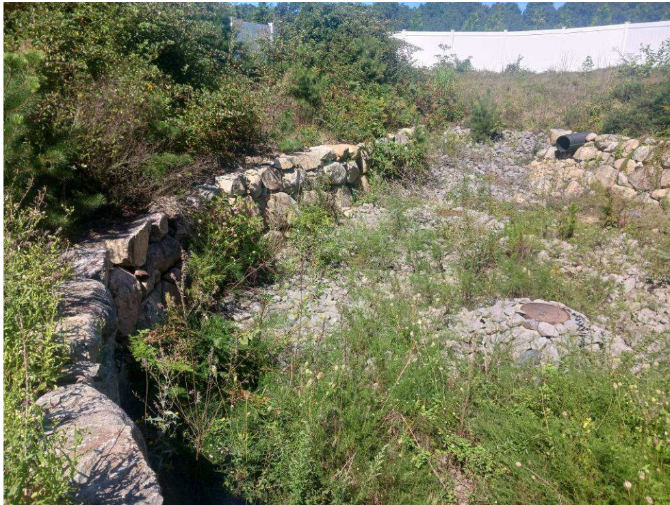
Figure 7 – Infiltration Basin Floor (dry)
