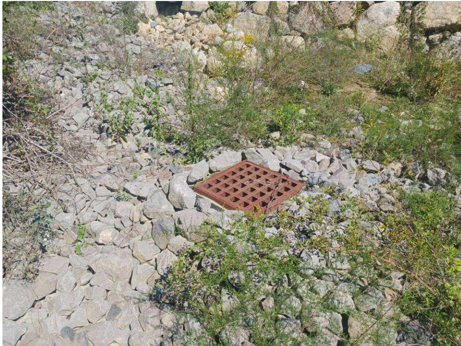
Figure 9 – Infiltration Basin Floor (dry)
