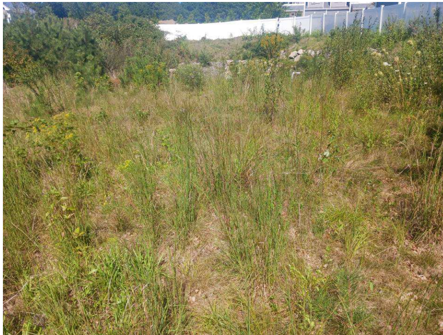
Figure 6 – Infiltration Basin Floor (dry)
