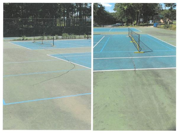
The Clarke Field Basketball court is similar to the adjacent tennis courts. The surface is cracking and there is 214 linear feet of cracks that require repair. The asphalt is the same age as the tennis courts and is failing but still worth rehabilitating and the Town should expect to get another five years from it after refurbishing. The 2021 budget pricing cost to rehabilitate this basketball court is \$25,000.
