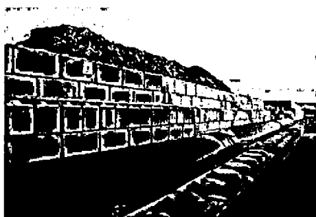
Negative air pipe connected to blower. Positive air biofilter in the background.
