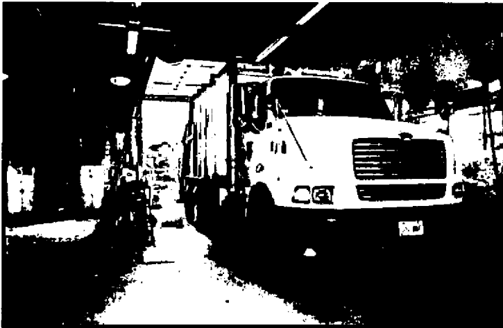
Only 1 1/2 vehicle maintenance bays for 4 Mechanics to maintain entire town fleet
