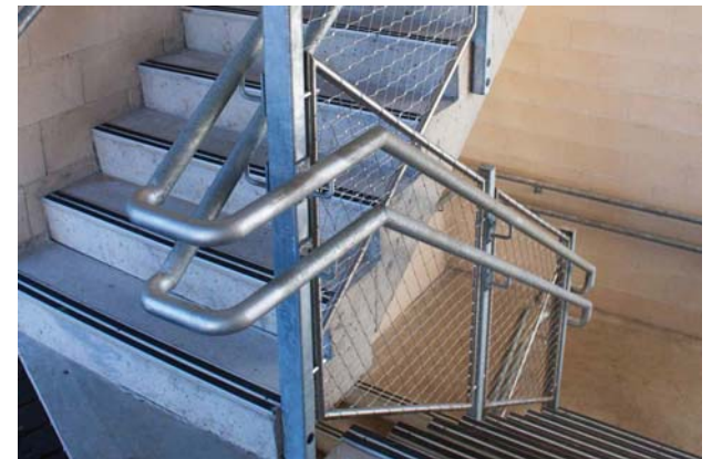
Mesh Guardrail Installed
