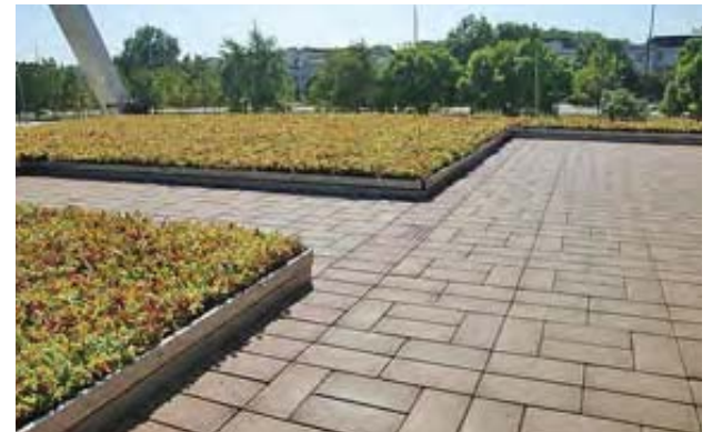
Roof Paver installed adjacent to sedum trays
