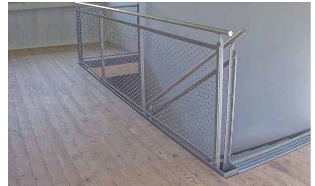
Mesh Guardrail Installed
