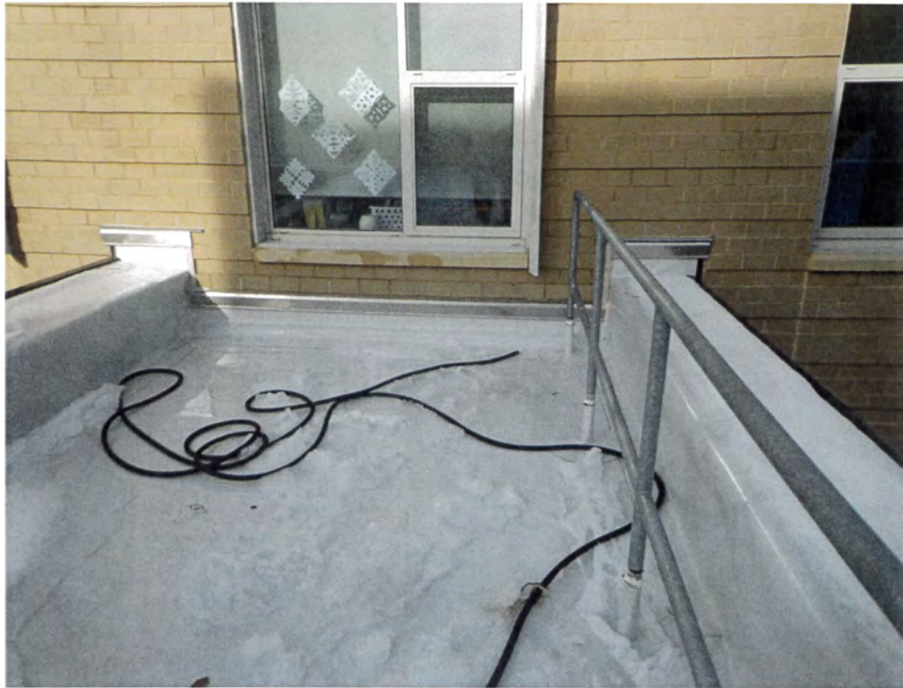
Photograph 1 Water Test 1 at Corridor Expansion Joint
