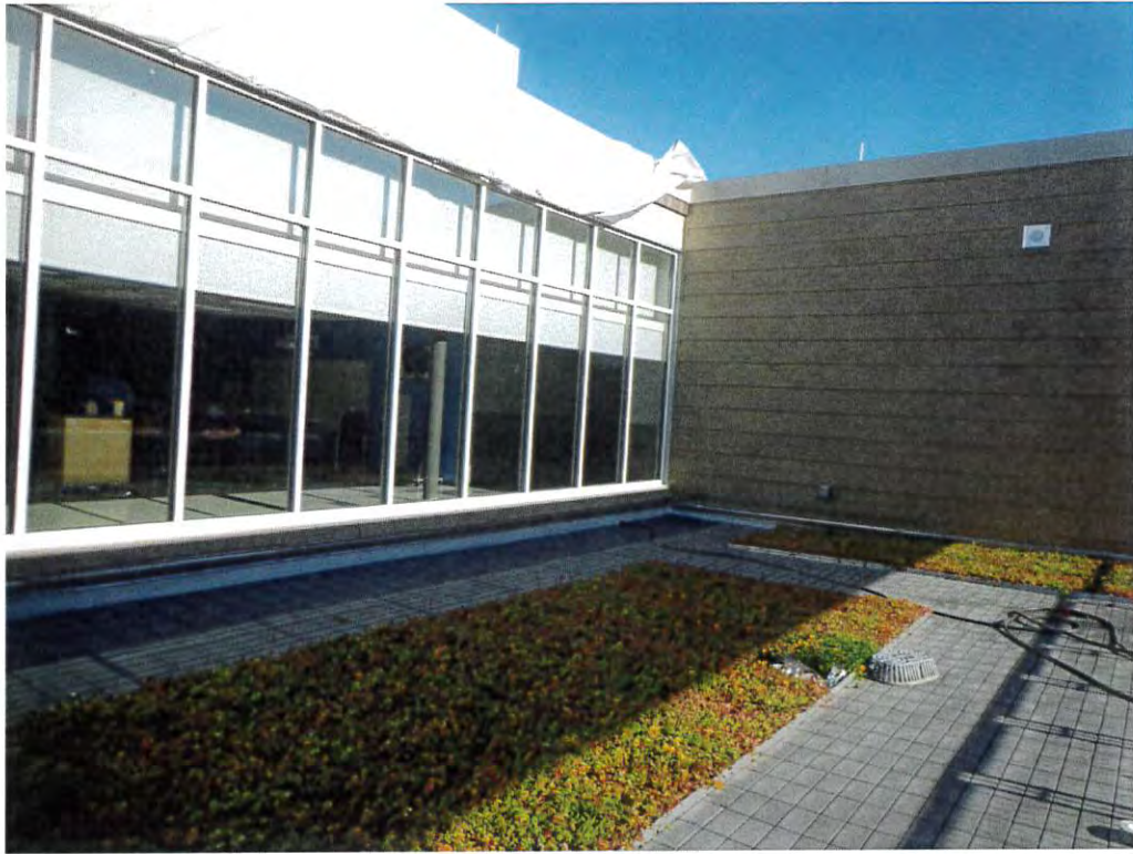
Photograph 3 General view of green roof
