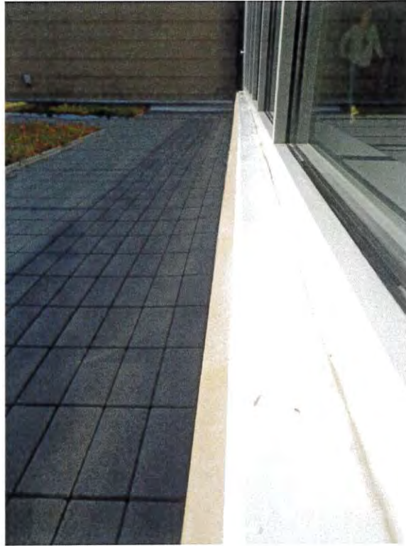
Photograph 7 Sill flashing at storefront window in Art Room
