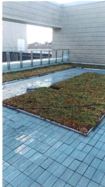
Photograph 8 Flood testing of green roof
