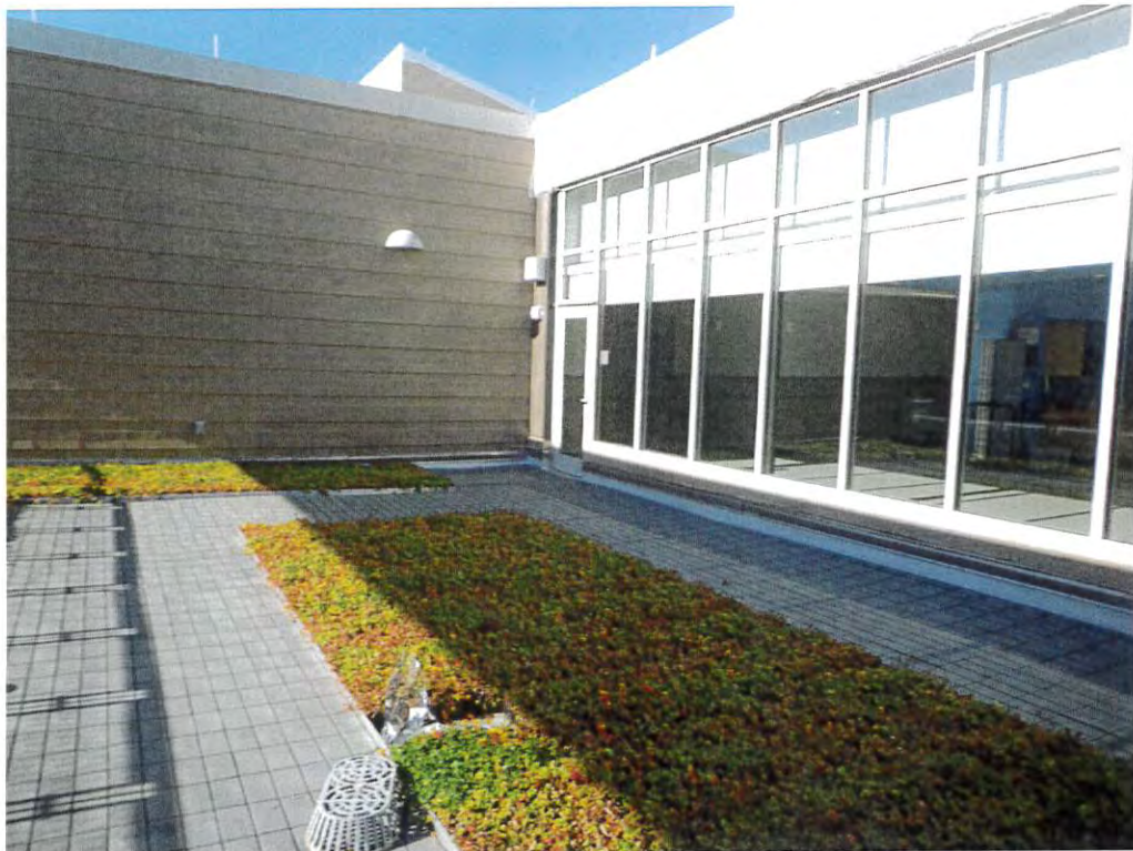
Photograph 4 General view of green roof
