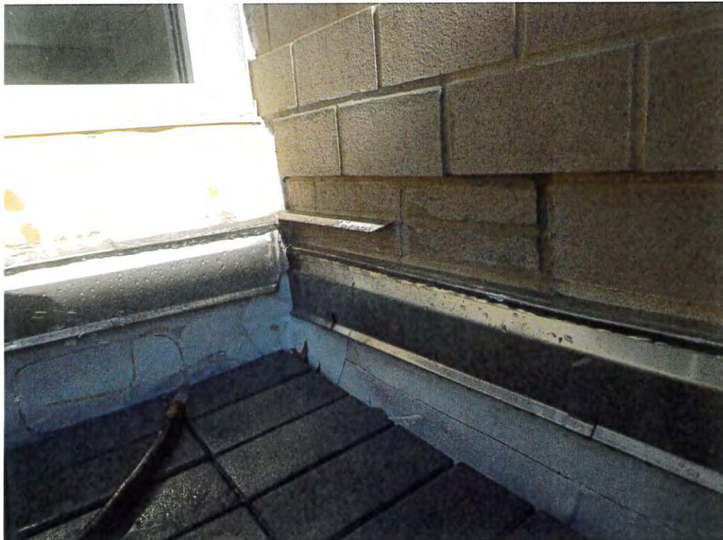
Photograph 6 Stainless steel counterflashing outside Art Room
