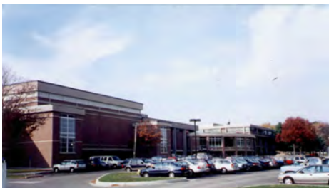
Westborough High School Westborough, Massachusetts Photo by DMBC
