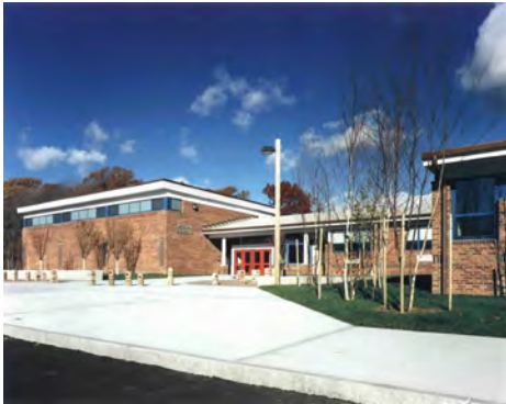
Brown Elementary School Natick, Massachusetts Photo by David Desroches
