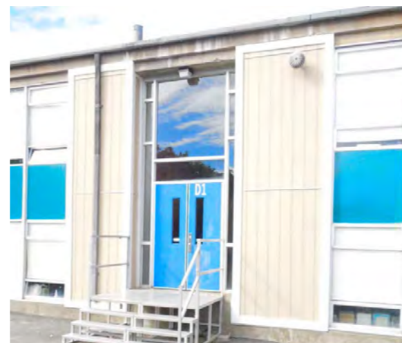
Panels Replaced at Addition
