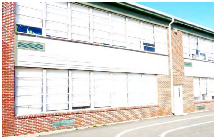
Vinyl Siding at Spandrel
