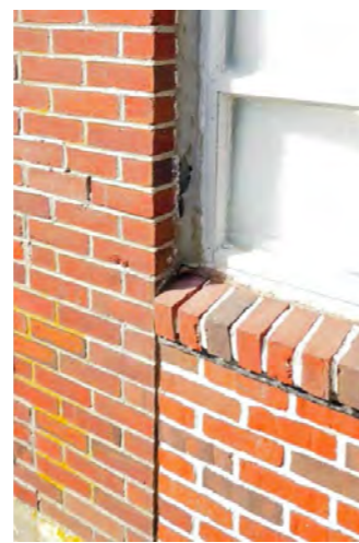
Caulking at Brick
