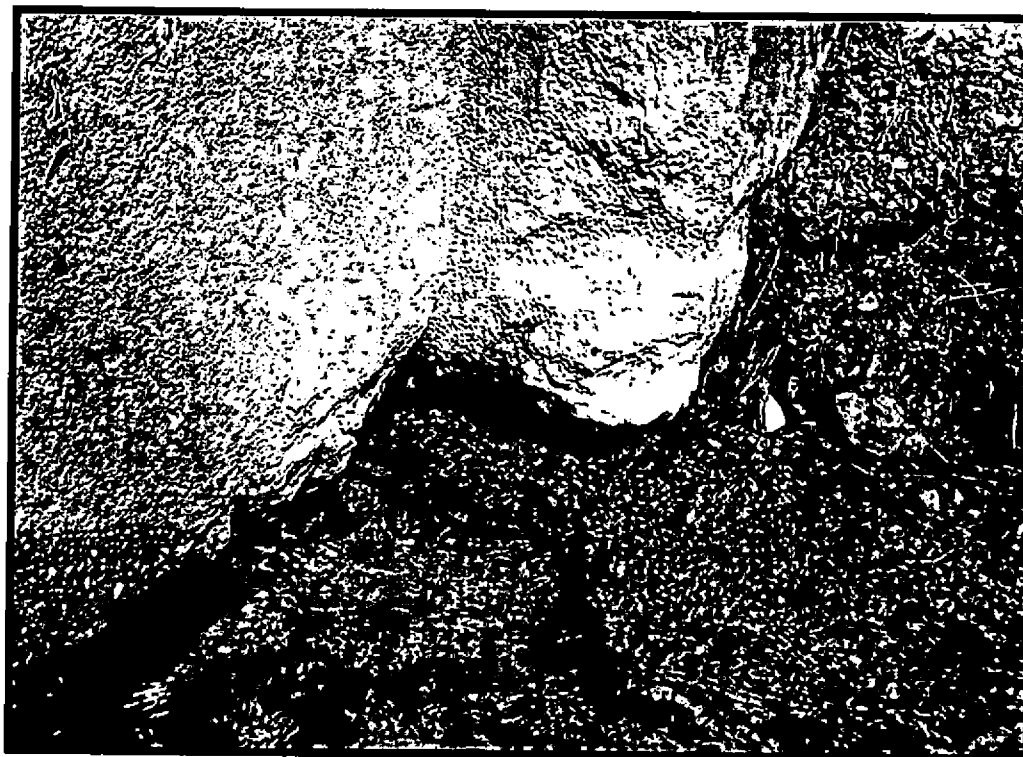
Photo 14. Tail Wall (South Face) Erosion & Undermining
