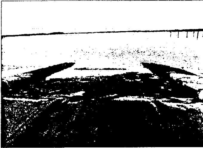
Bourne Town Ramps, December 8, 2014
