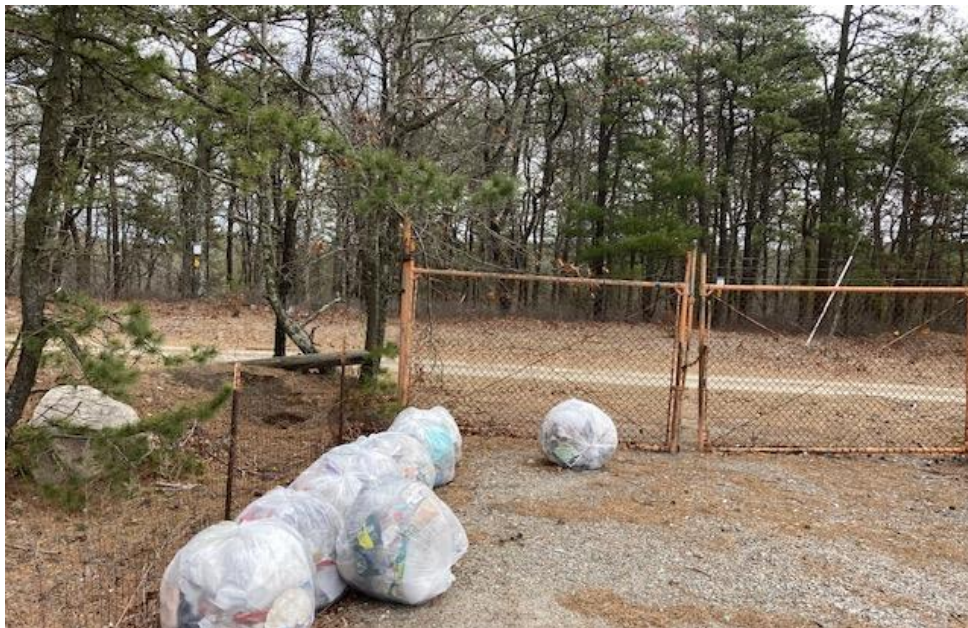
Photo 1. Wire grid fencing along the eastern property line extending from the access gate to the perimeter road within Joint Base Cape Cod.
