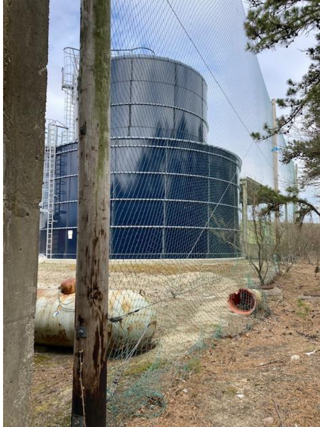
Photo 2. Litter fencing located along the eastern boundary of landfill operations.
